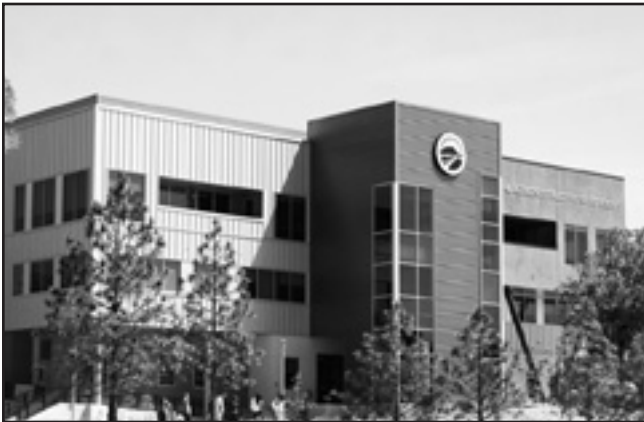
Student and Administrative Services building, (SAS)
