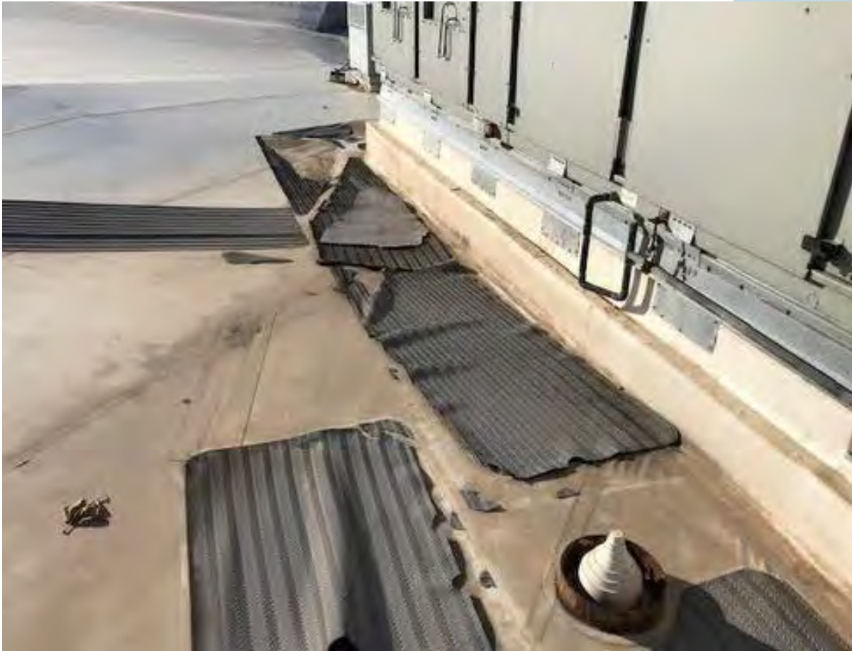
Media Center Roof
