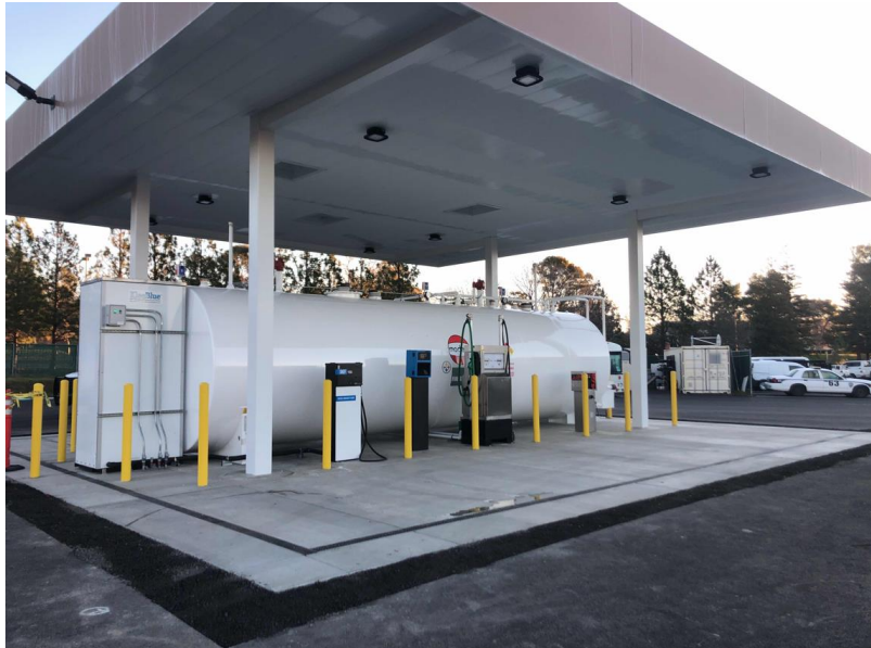
Underground Storage Tank
