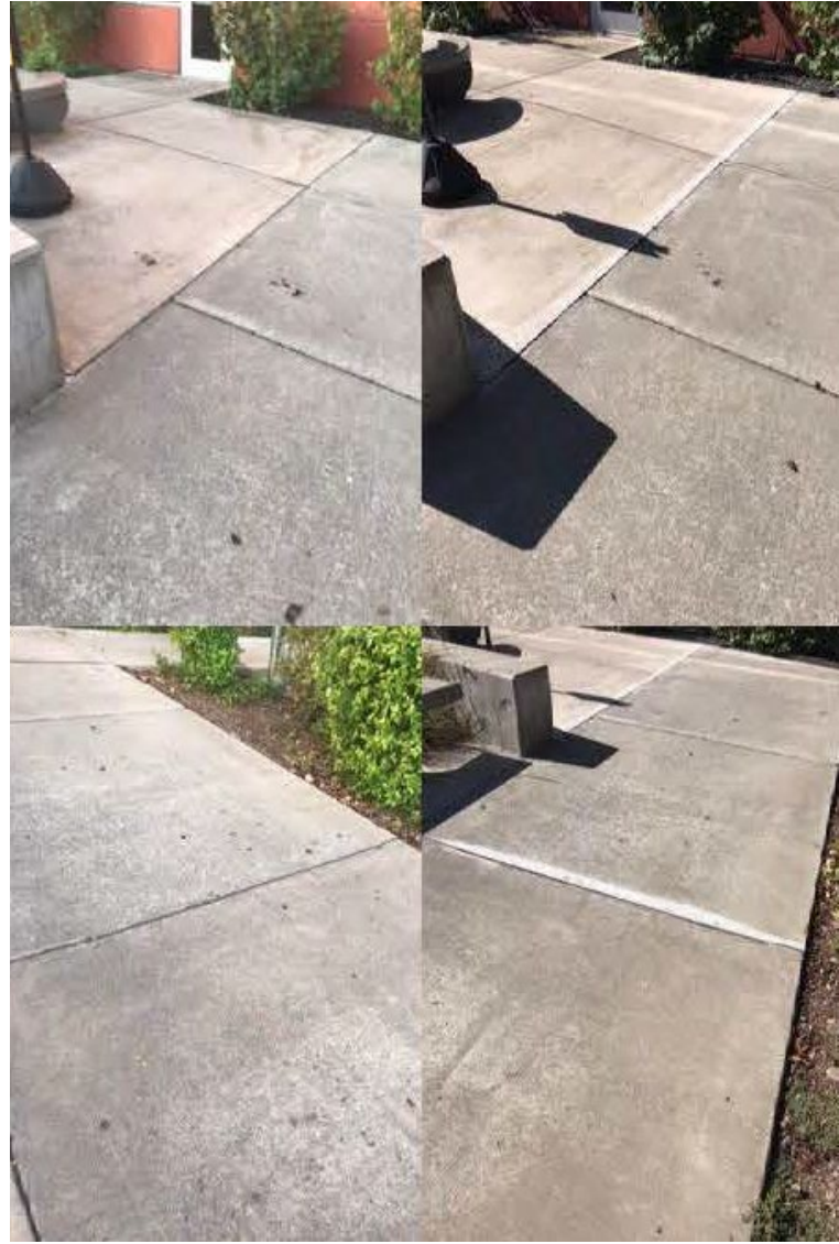
Sidewalk Trip Hazards Repair
