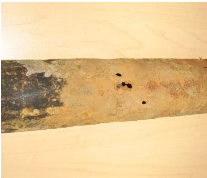
Section of gas pipe recently replaced
