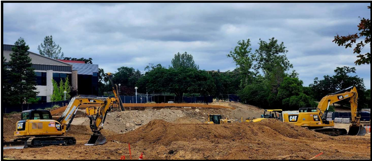
Demolition and site work for Science building
