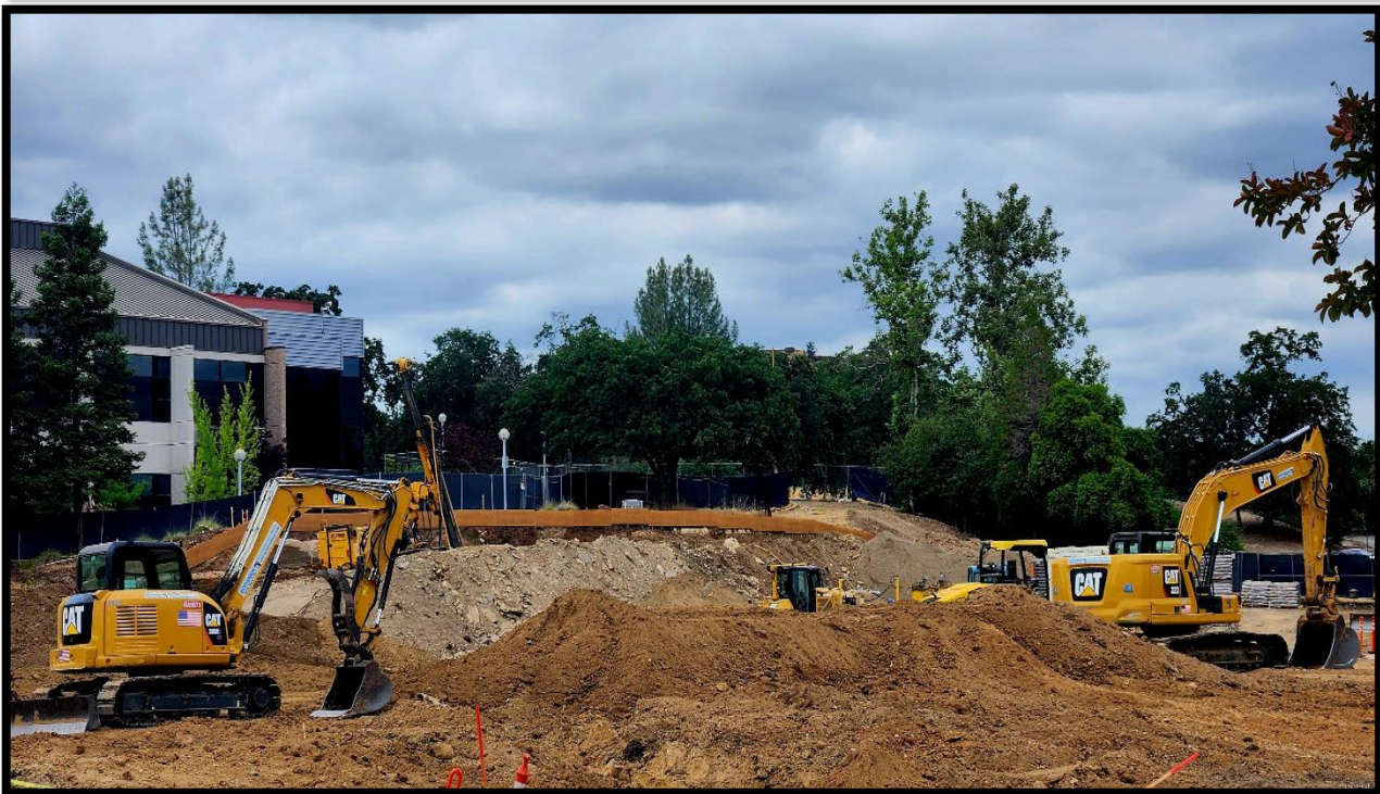
Demolition and site work for Science building
