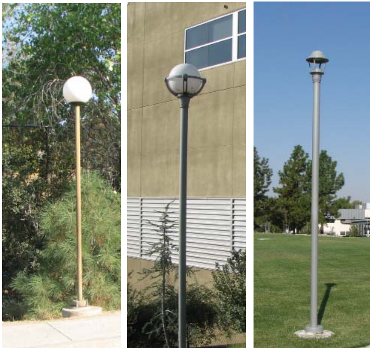
Three styles of walkway lighting on the main campus
